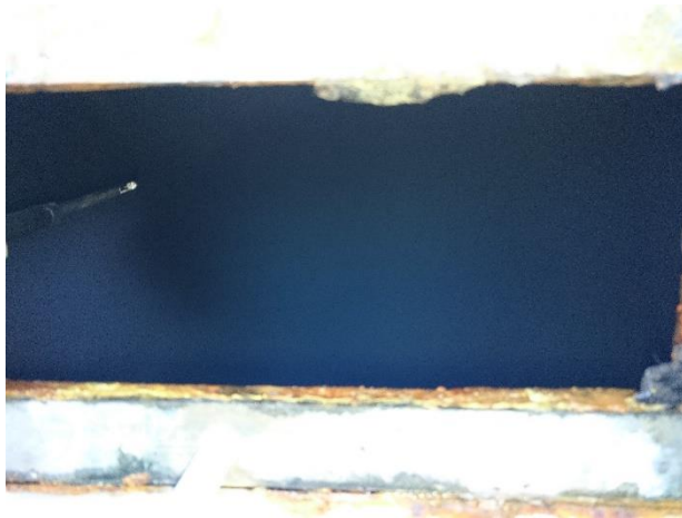
Inside of FGD outlet duct
