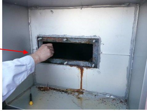
Cut the hole to the duct and welding flange
