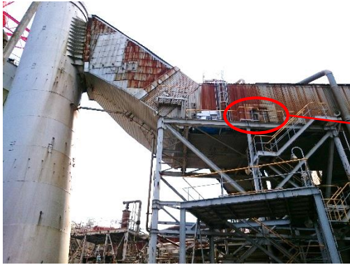
Cut the hole to the duct and welding flange
