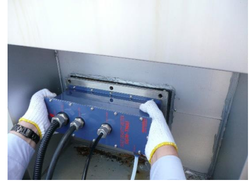
Attach the detector to the duct
