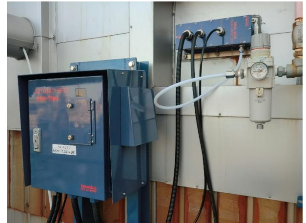
Zero & Span adjustment and set heater temperature of DDM-TMA1
