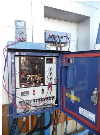
Zero & Span adjustment and set heater temperature of DDM-TMA1
